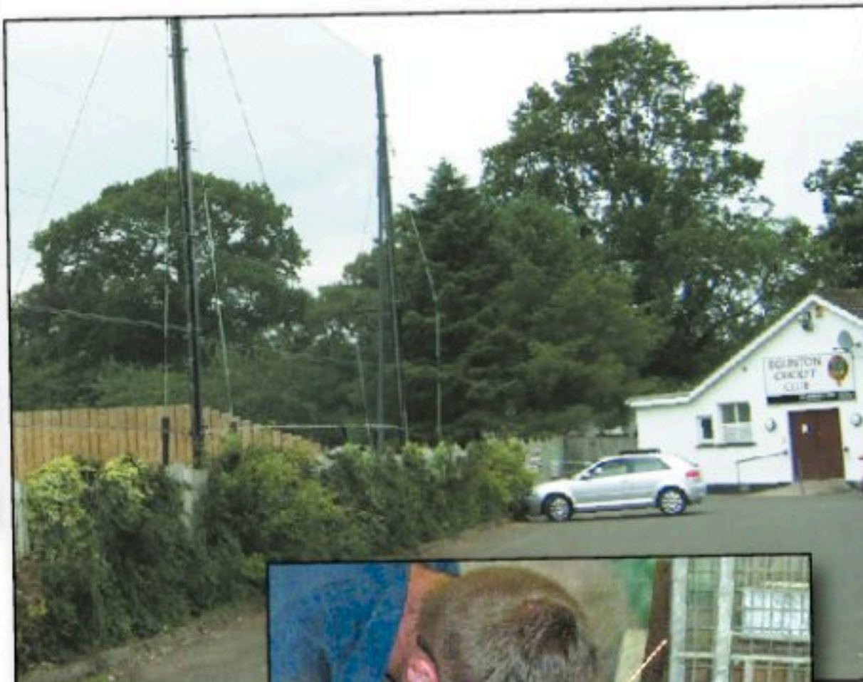
■ SAFETY FIRST: At Eglinton Cricket Club, the car park is protected from stray cricket balls, with Specialist Fencing Contract's 12 metre high and 80 metre long netting and upright system. FW-2B.
