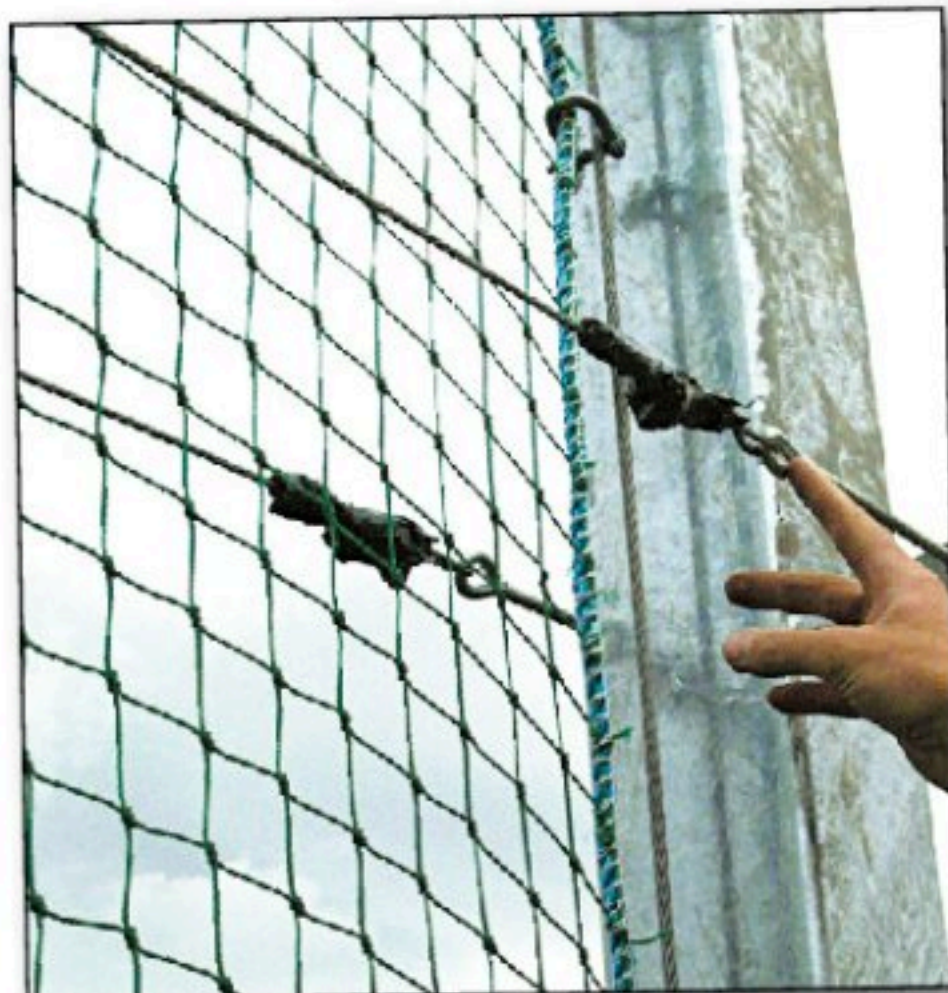
■ TWIN WIRE: A patented solution involving the use of high tensioned double wires with a 'floating net' in-between to secure 'ball stops', was designed by Eamon Scullion of Specialist Fencing Contracts, Ballyscullion, Bellaghy. FW-1S.
