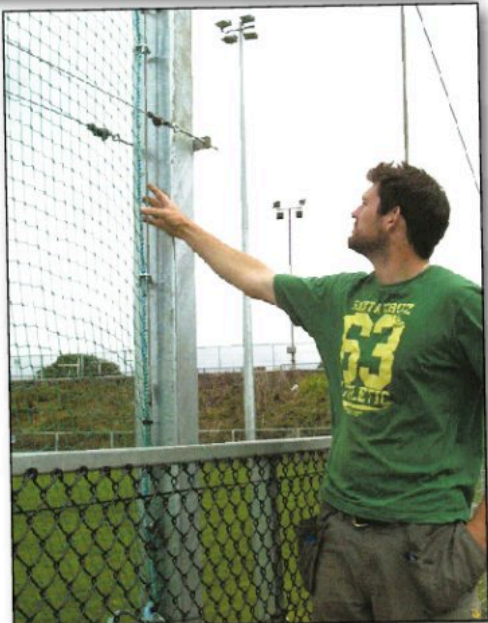
■ FLOATING NET: Dominic Scullion points out the simple yet ingenious solution to flapping and sagging 'ball stop' nets; a 'floating net' designed and patented by Specialist Fencing Contracts, Bellaghy. FW-1R.
